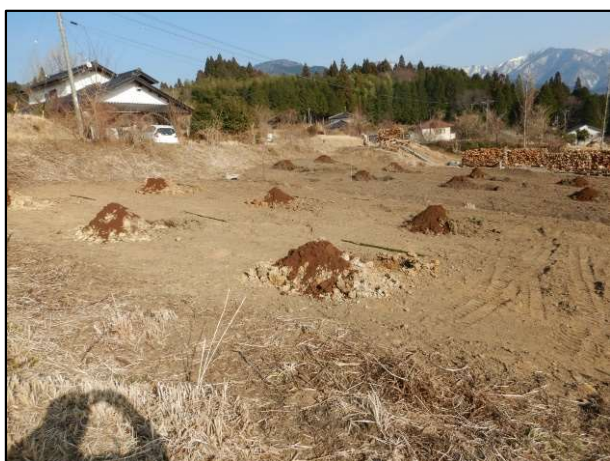
[植栽場所を掘削]
